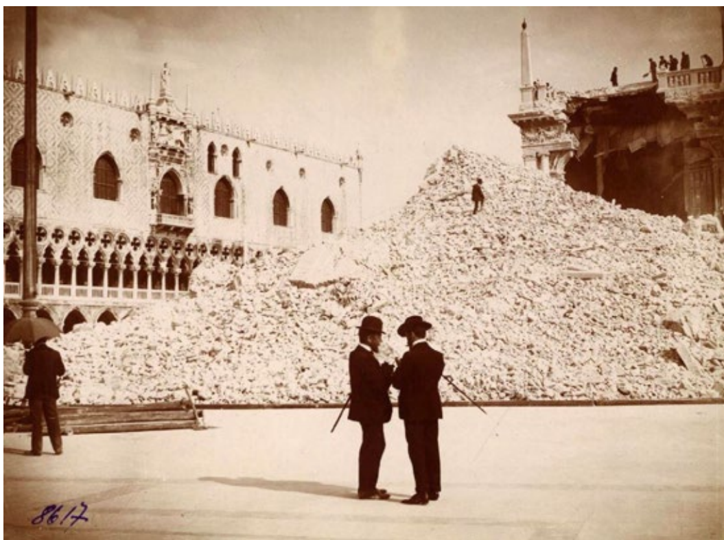
Piazza San Marco in Venice after the collapse of the Campanile (1902)
